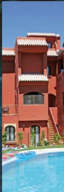
PRIVATE HOUSES AND BUILDINGS
